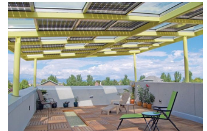
Usable Rooftop Space allows for recreational opportunities. Credit: [22]
